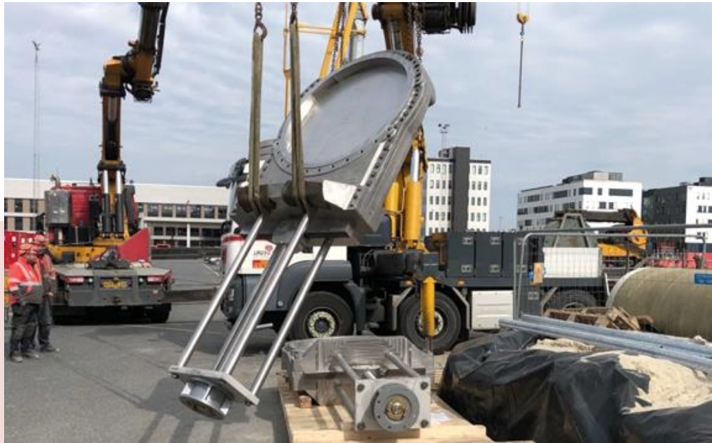
Delivery of one of the DN 1200 Wey knife gate valves without actuator
