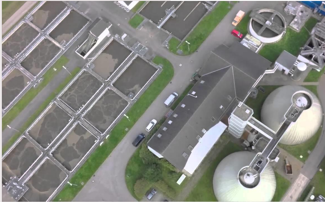
The municipal wastewater treatment plant in Baden-Baden•Sinzheim Photo: City of Baden-Baden
